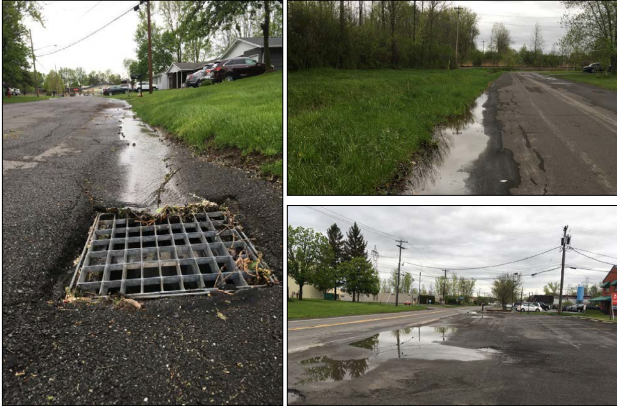
Photo 15: Various examples of existing stormwater management conditions throughout the town. Minor puddling as pictured here may create ice hazards in winter. Furthermore, informal roadside drainage compromises the safety of roads for all users, regardless of mode. Many recurring flooding events could be mitigated with comprehensive flood planning and infrastructural improvements.
