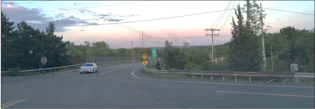
Photo 8: The Kinne Road Bridge provides a narrow sidewalk on its northern side that pedestrians can use to cross over Interstate 481; however, they must compete with heavy and fast paced traffic. View looking east from the bridge's western end.
