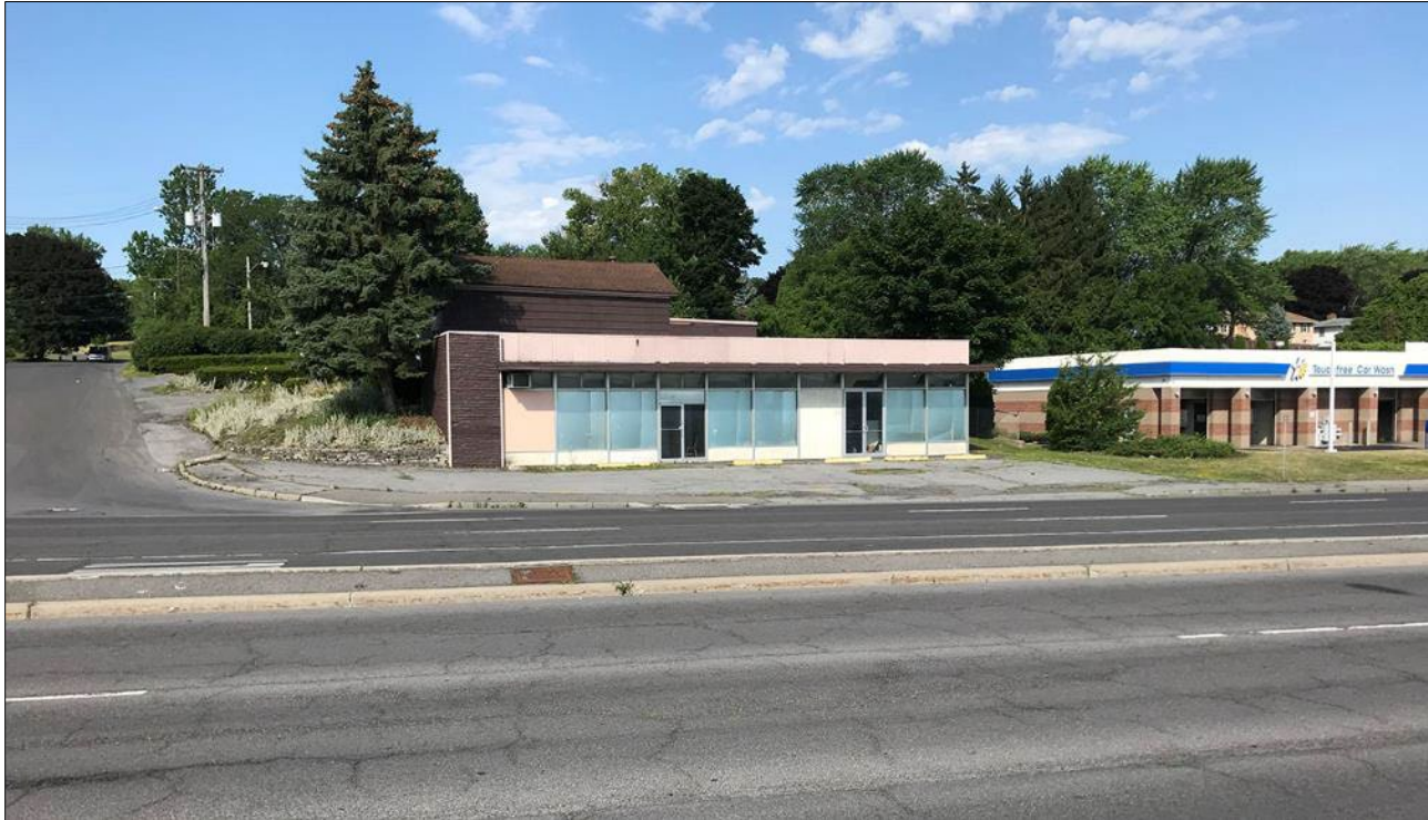
Photo 6: Abandoned commercial building located at 3350 Erie Boulevard; view looking west from across Erie
